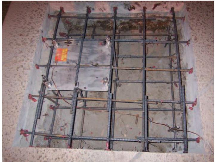
1. Remove 1 nut from each anchor insert. Place the anchor inserts through the larger hole of the anchor jig plate. Thread the removed nuts back onto the anchor inserts. The anchor plate should be sandwiched between the two nuts on each anchor insert. **SEE SECTION D-D**
